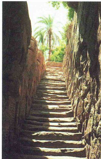
BELOW The steps of the Nilometer on the island of Elephantine at Aswan measured the height of the Nile. This example dates to the Roman period. (P. T. NICHOLSON)
