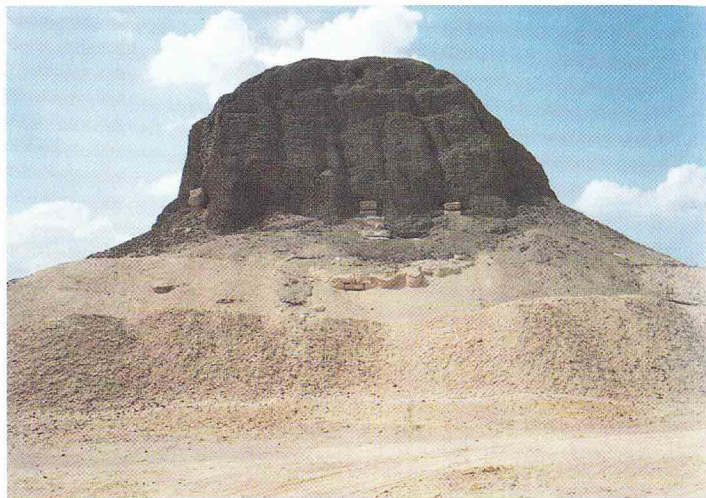
The pyramid of Senusret II at el-Lahun is constructed of mud-brick around a series of limestone walls, some of which can be seen at the base of the pyramid. The structure has lost its outer casing and so has weathered to a rounded profile. (P. T. NICHOLSON)
