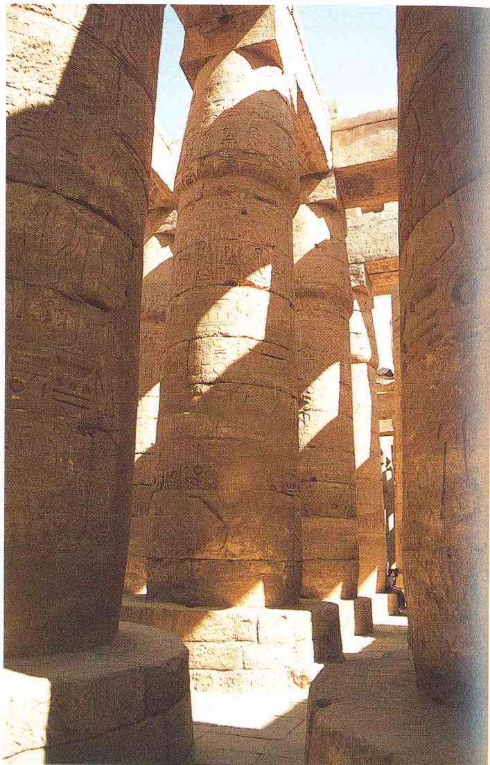
Part of the Great Hypostyle Hall of the temple of Amun at Karnak. These are the smaller, closed papyrus bud columns: the open papyrus columns along the axial route stand 23 m high.
