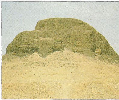
The pyramid of Senusret II at Illahun has a mud-brick core surrounded by the remains of a limestone casing.
